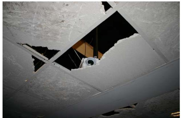
Fig. 2: Projector placed above the ceiling.
